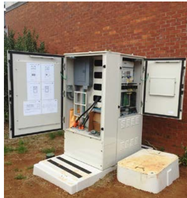
The Adtran Total Access 5000 fiber access platform installed within an environmentally hardened cabinet.
